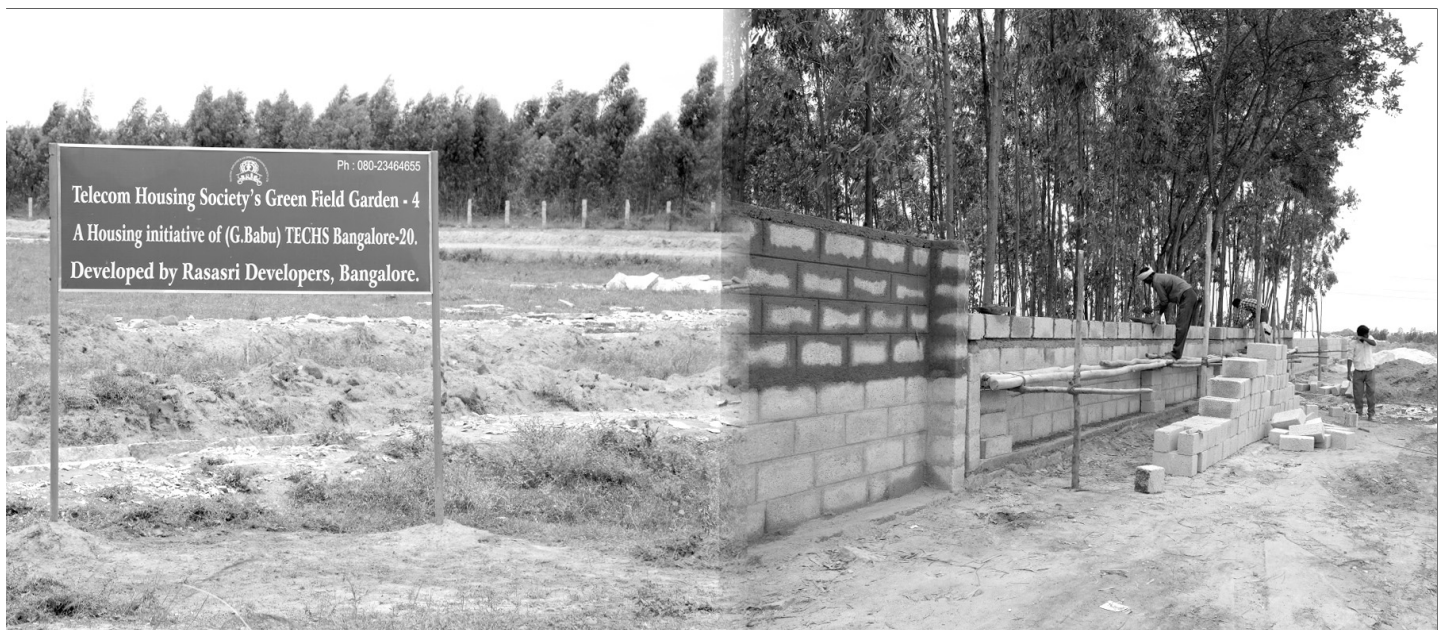
Work Under progress of GFG 4 Layout
